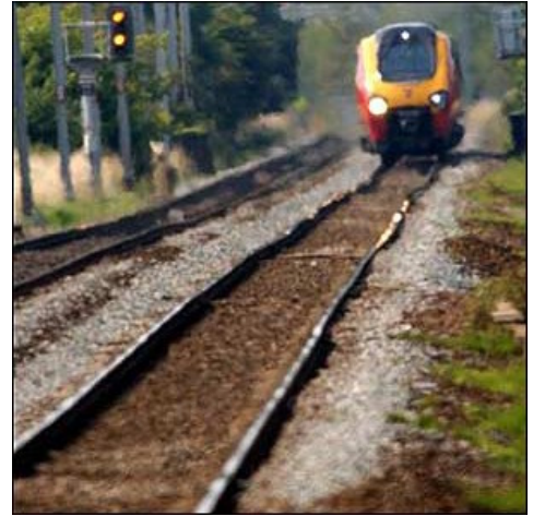
Soaring temperatures in the summer of 2003 forced rail networks to be closed because the track buckled in the heat. (Courtesy BBC).
